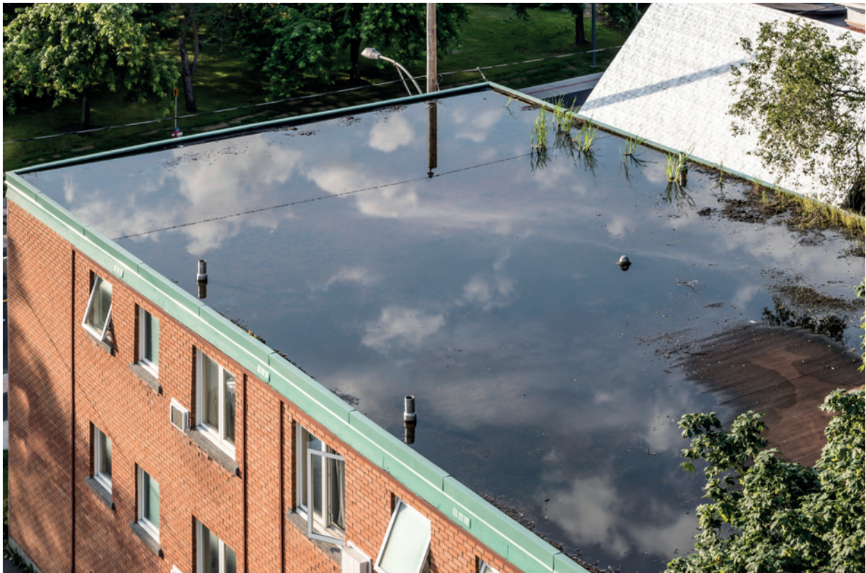
Figure 1: Ponding on a typical flat roof
