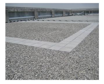
Local Firestone Master Contractor Western International recommended the use of the RubberGard EPDM membrane due to its compliance with ESTIDAMA requirements, its long-term durability - even in the extreme UV radiation and heat of Abu Dhabi- and its capability to meet the fast installation rates that were set for the construction of the Yas Mall. In total, about 100,000 m² of 1.5 mm thick RubberGard EPDM membrane were used in this project.
